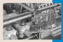
Dwarfed by the machine, Jim Buchwald stands near this 600 rpm, 100,000 lb. rod load compressor in 1966 that helped get him started in the compressor business. The Enterprise design was the fastest compressor of that size ever produced until the advent of the JGB compressor in the late 1990s.
